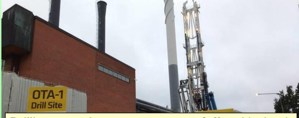
Drilling costs increase <u>exponentially</u> with depth Heat in the rock increases <u>linearly</u> with depth So there are severe limits to EGS depth
